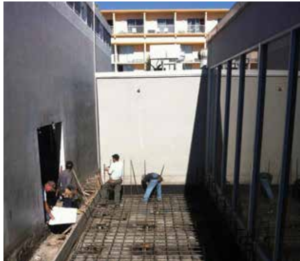
AFTER THE HELICAL PILES ARE INSTALLED AND CAPPED, REBAR IS ADDED FOR REINFORCEMENT PRIOR TO POURING CONCRETE
