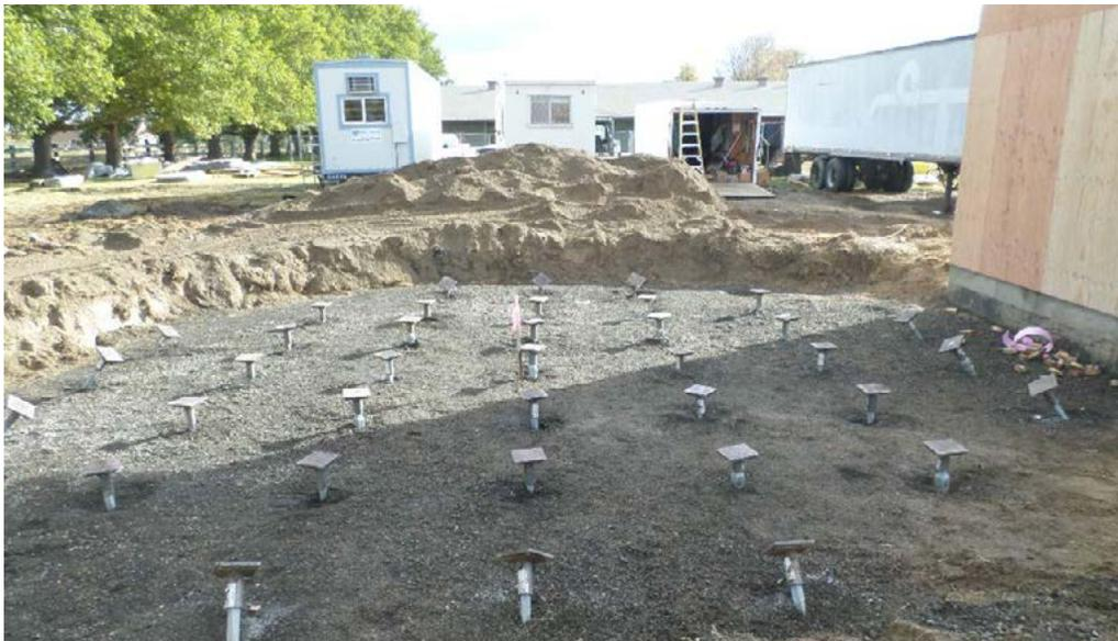
Montana Helical proposed an alternative solution utilizing CHANCE® Helical Piles. From a material standpoint and given the anticipated depth, helical piles are less expensive, utilize smaller equipment, provide faster installation and the material is readily available.
